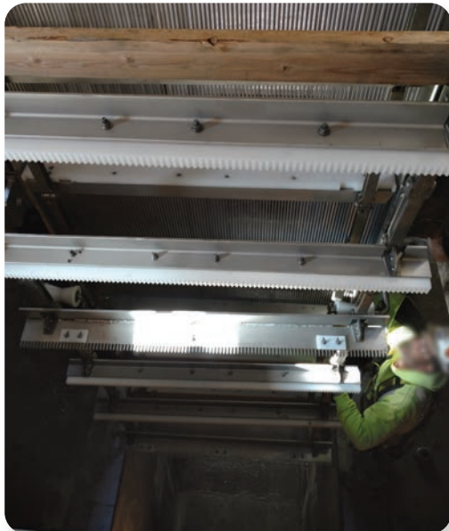
Lock Link screen arrives fully assembled or with bolted modular pieces for deep channels.
