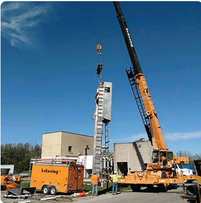
Lock Link Screen Installation New Castle Indiana
